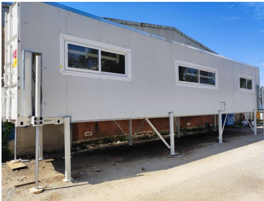
Figure 4. General external view of the prMRF, showing side windows, the hydraulic legs for lifting and the static legs enabling the elevated operation of the container.
