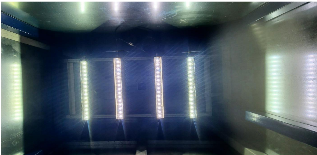
Figure 1: The setup installed by ROBENSO at HERRCO's MRF for mixed waste sorting. Top image shows the dark room in place, above the MRF conveyor. Bottom image shows inside the dark room, the lighting and camera setup used for taking RGB images (bottom to top view).
